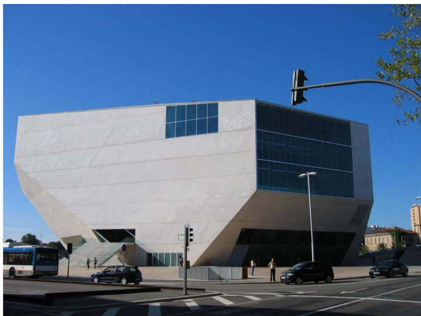
The initial concept was for a translucent building with a metallic structure. Cost reasons and the loss of the transparency effect, which was the inevitable result of the structural elements’ density, led to the choice of white concrete. Although it clearly appealed to Rem Koolhaas, white concrete had not been proposed initially because it is not a common material in Northern European countries where it is difficult to find skilled labour to carry out top quality work in exposed concrete.
