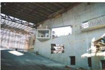
The acoustic isolation of the main auditorium is done by means of separating this from the rest of the structure. This separation is referred to as being a “box within a box”. In this separation the floor, walls and ceiling of the auditorium only come into contact with the building’s structure through resilient mounts.
