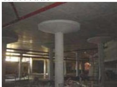
The car park layers are massive reinforced concrete slabs. They are supported on isolated pillars, on reinforced concrete walls, on the sloped walls of the auditorium building, and on the peripheral retaining walls.
