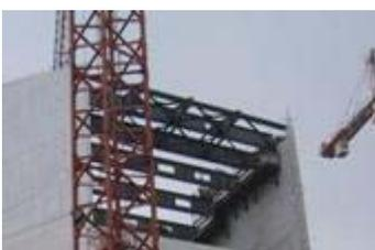
Due to the slight slope of the roof panels, certain free edges which were to be very slender would have had excessive deformations unless the reinforced concrete shell had not been replaced by steel structures comprised of open-web girders or beams in a welded, variable cross section
